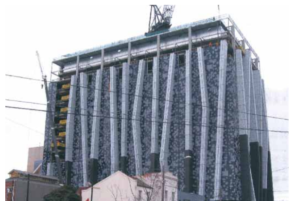
Construction at 198 Berkeley Street is almost complete
